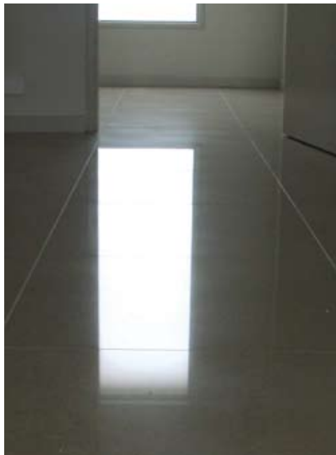
Photo No. 11. The same area after de-glossing and re-glossing treatment. Note only the 4 tiles out from the doorway were treated as a test to meet customer satisfaction.
