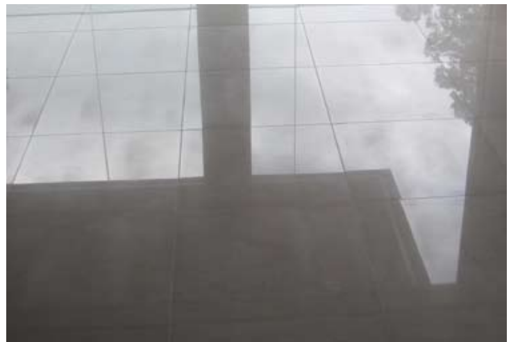
Photo No. 4 , in the same room as photo No. 3 shows a typical complaint of "shadowing" in the reflected light
