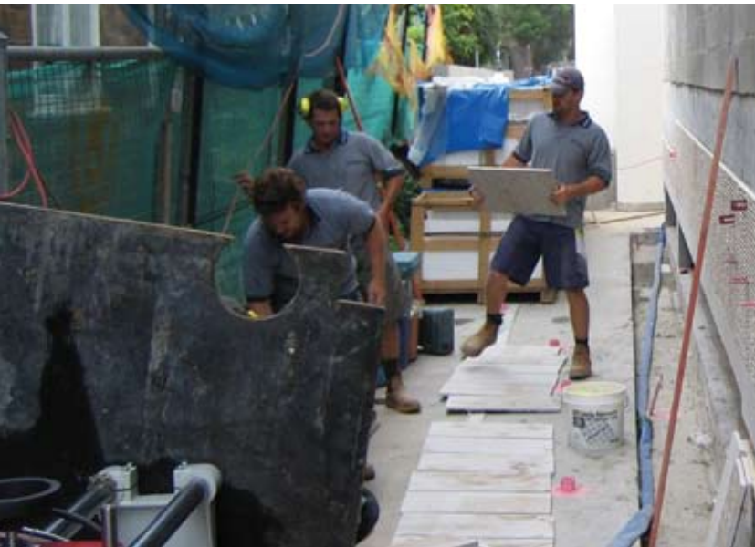
Above: The cladding was applied to the surface of core-filled concrete block masonry using Latapoxy 310 adhesive. Right: Brackets are used to take up spans greater than 20mm. Below Left: A second granite façade completed with Latapoxy 310.
